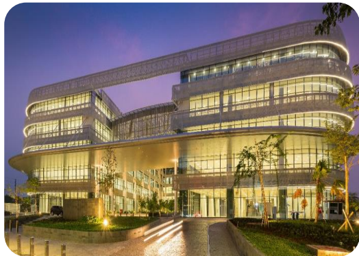
Green Office Park1 BSD
